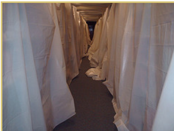
The stacks on the fifth floor were covered (as a preventive measure) and the area restricted to staff only for the duration of the roofing project
